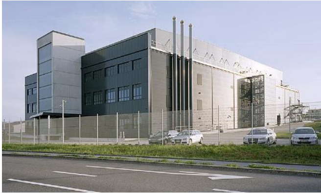
E-Shelter Rümlang (Tier-4)
